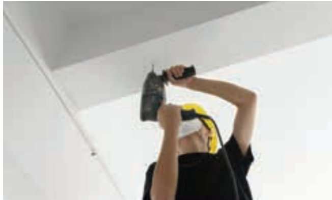
5. Drill at the marked position with a percussion drill, and fix the interconnected profile onto the wall
