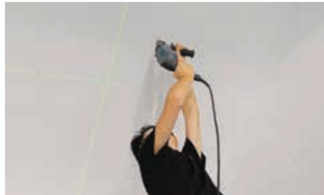
4. Drill at the marked position with a percussion drill, and fix the connector of one end of the pendant cable to the hole.
