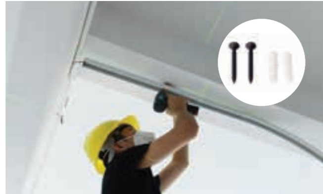
5. Drill at the marked position with a percussion drill, and fix the interconnected profile onto the wall
