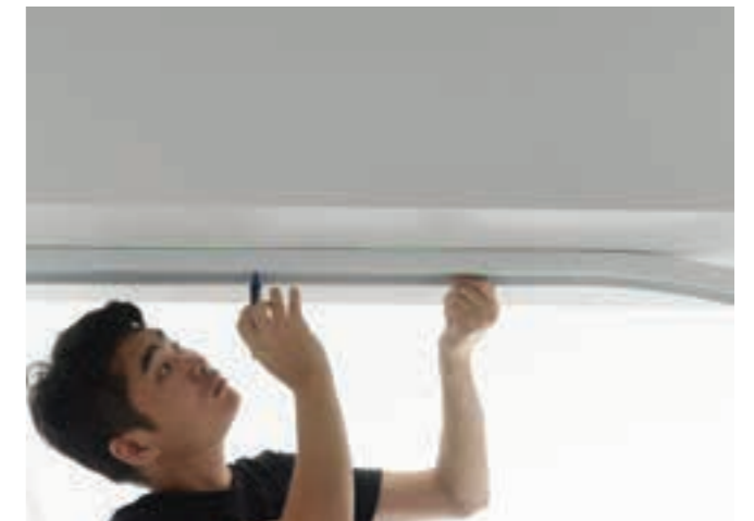
4. Use a gradienter to determine the drilling position of profile installation on the ceiling, and mark with a marking pen
