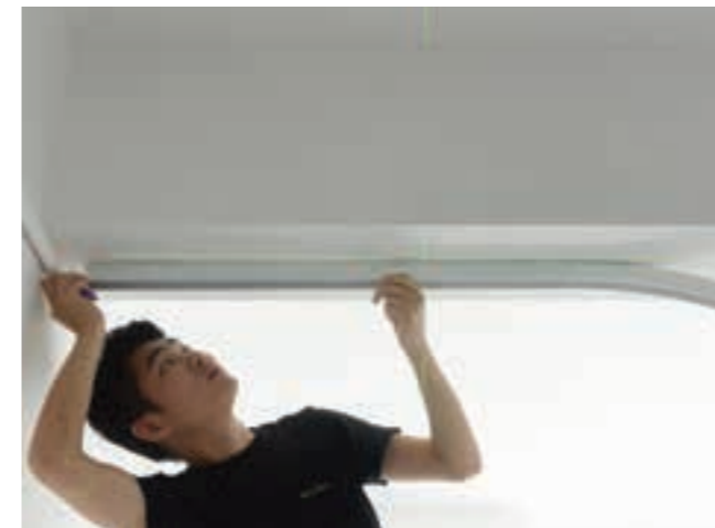
4. Use a gradienter to determine the drilling position of profile installation on the ceiling, and mark with a marking pen
