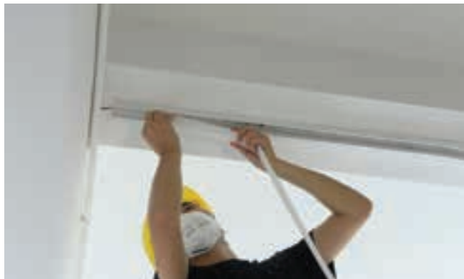
7. Mount the diffuser into the luminaire slowly, and power on to light up the luminaire
