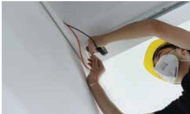
6. Power on to test the luminaire, and install the diffuser if it works well
