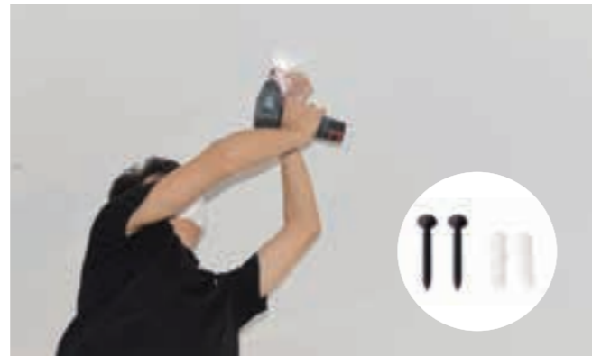
4. Drill at the marked position with a percussion drill, and fix the connector of one end of the pendant cable to the hole.
