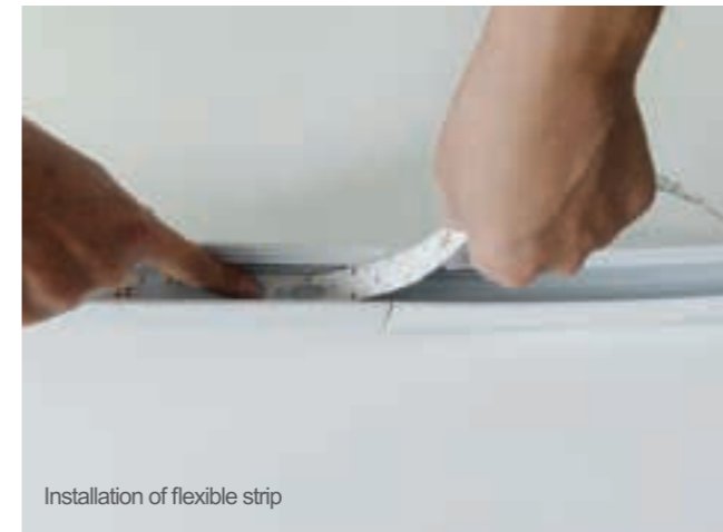
3. Mount the light source into the profile (installation details are referred to in Page9)
