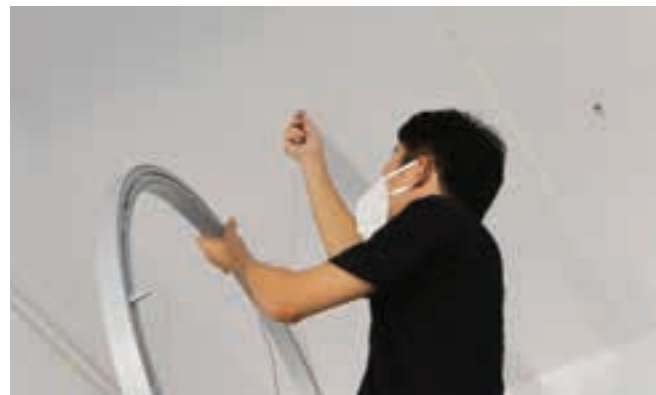
5. Connect the prepared pendant cable of the luminaire to the connector on the ceiling, and adjust the height of the pendant cable and remove the surplus part.
