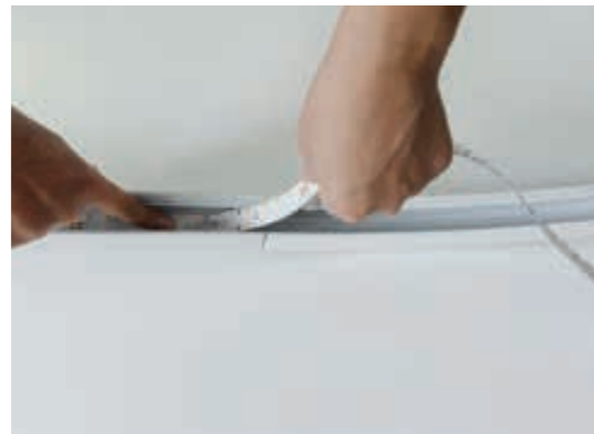
Paste it properly according to the length needed
